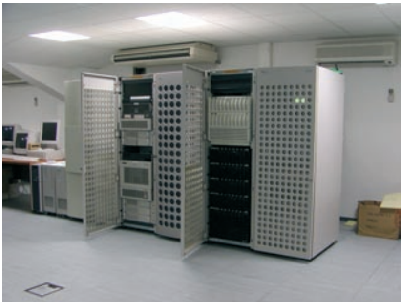
Important CSSA working places, equipped with state-of-the-art technology
